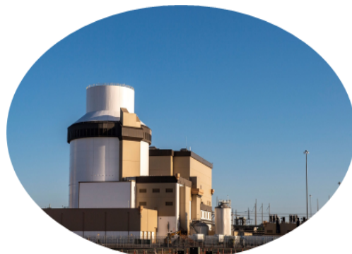
Westinghouse AP1000 1100MW
