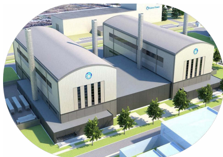
Kairos Power KP-FHR 140 MW
