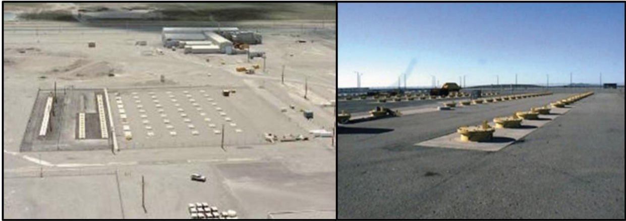
Figure 24: Dry cask storage of Fermi-1 SNF at the INL's Idaho Nuclear Technology and Engineering Center. 1st-generation underground vaults built in 1971 (left) and 2nd-generation underground vaults built in 1984 and 1985 (right). 84
